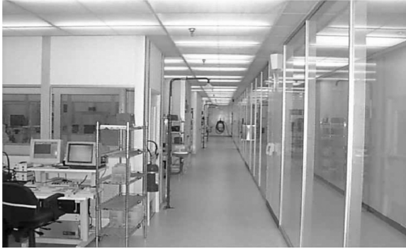
6,500 square foot Class 100 wafer fabrication clean room.
